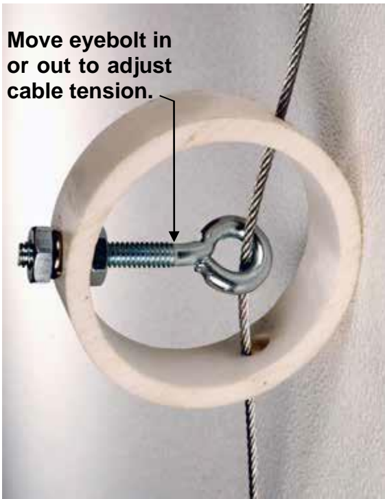
(Cable Adjuster Assembly)
